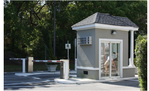
Wild Dunes Access Control Gate Installation.
